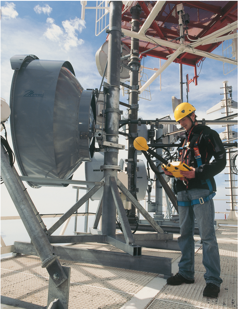
Figure 1: SRM-3006 in on-site use
