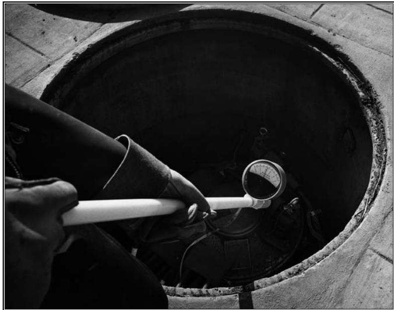
Figure 3: Application of voltmeter probe for line to ground voltage measurement on voltage test point.
