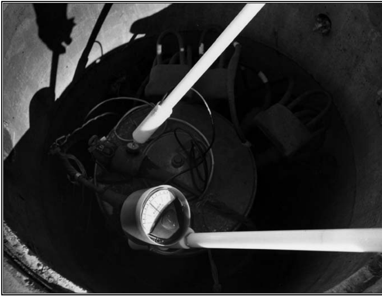
Figure 4: Application of voltmeter probes for phasing or line to line measurement on voltage test points.
