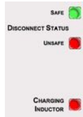
Figure 11 - Disconnect Status & Charging Inductor LEDs
