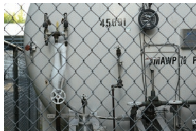
Difficult inspection sites
