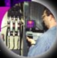
Connection problem on 200 Amp fused disconnect
