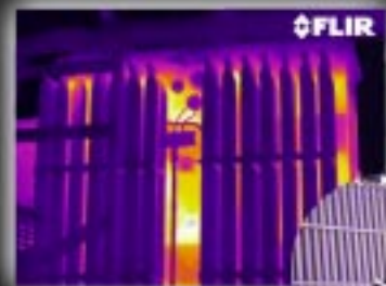
Plugged cooling fins on 13.8KV transformer
