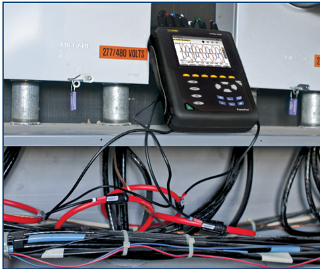
AmpFlex® flexible current sensors facilitate easy access to current carrying conductors.
