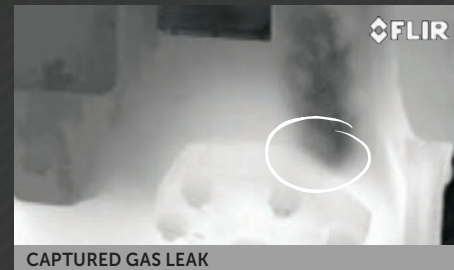
CAPTURED GAS LEAK
