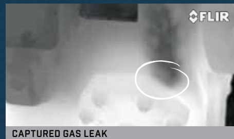
CAPTURED GAS LEAK
