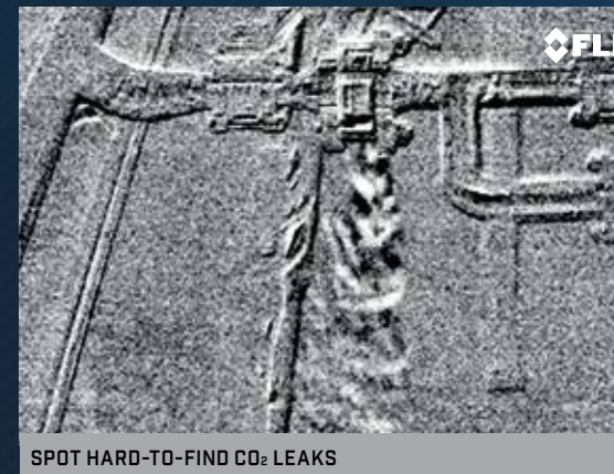
SPOT HARD-TO-FIND CO 2 LEAKS
