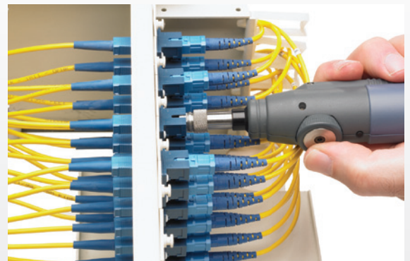
Patch panel bulkhead inspection
